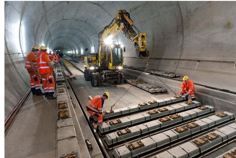
Underground tunnel construction
